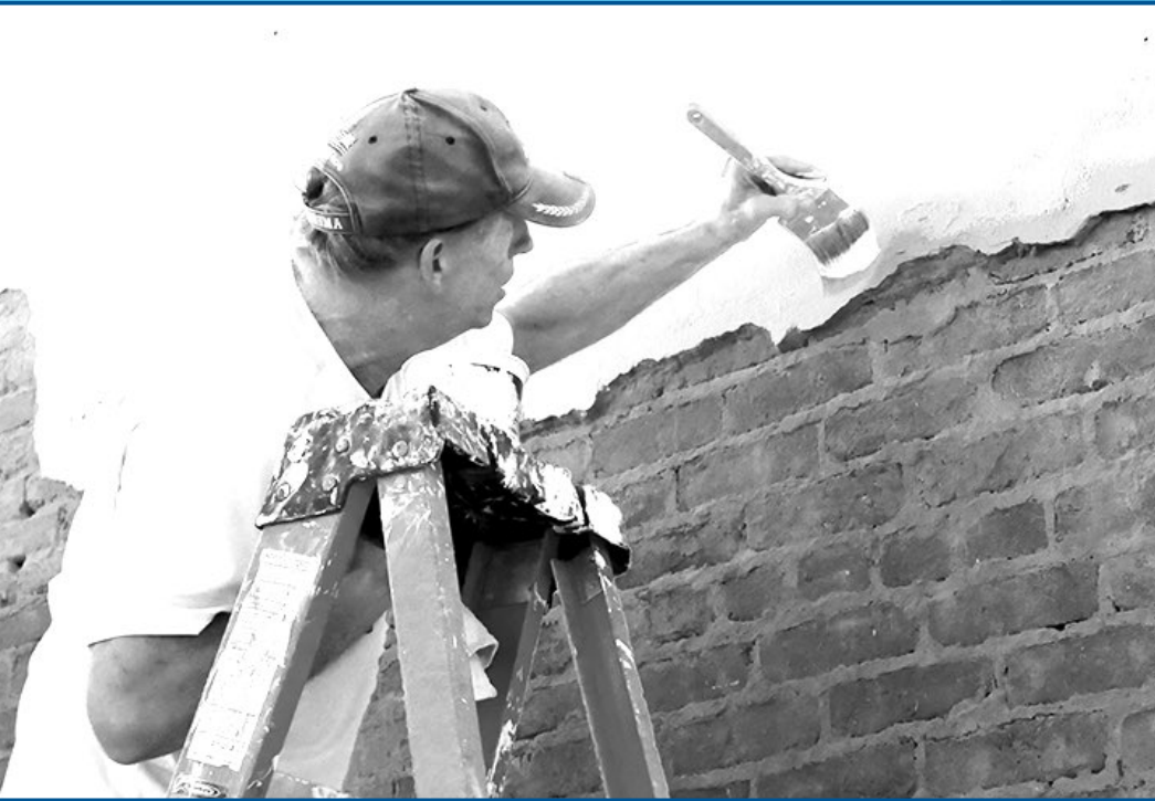
Michael Bednarski paints the plaster left in place on the exposed brick wall at the north end of the gallery.
